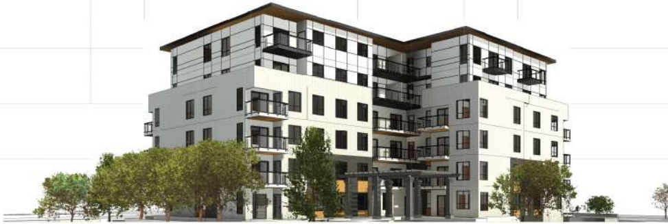
1 SOUTH WEST VIEW (REAR-SIDE)
