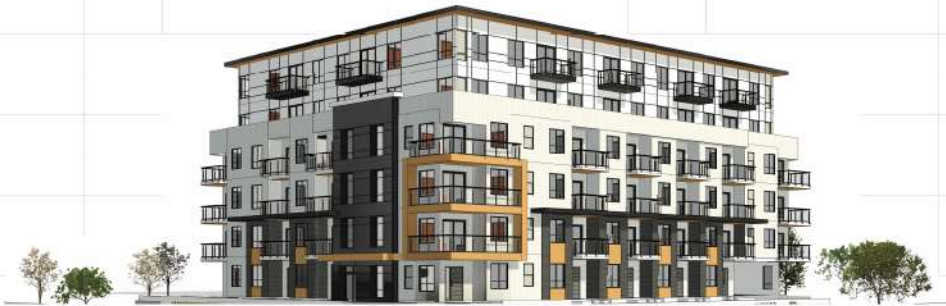
VIEW ALONG NORTH EAST CORNER
