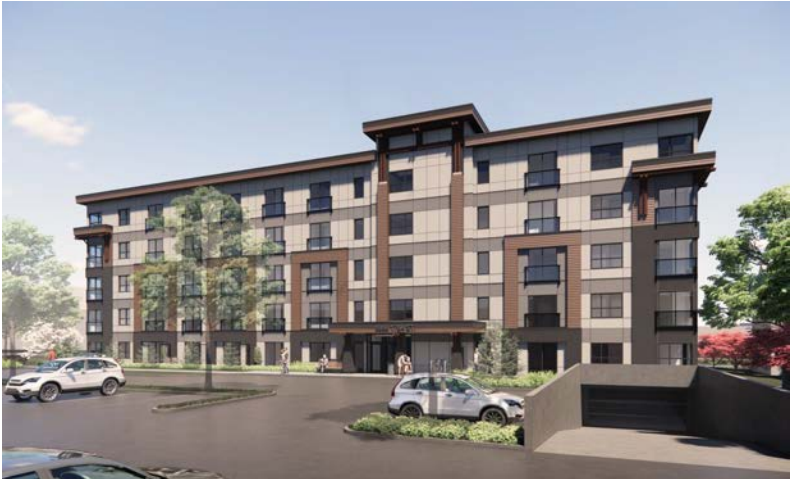
parkade entrance east side
