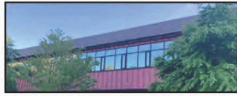
REFERENCE - SIMILAR TO EXISTING SLANTED ROOF
