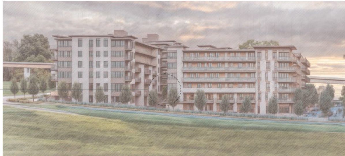
4 View from North [72nd AVE]
