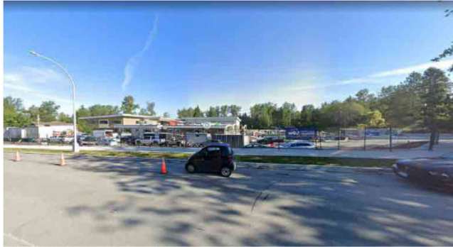
regent road elementary (under construction)
