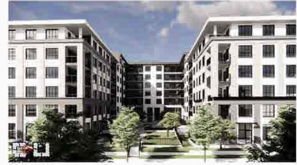
VIEW LOOKING WEST TOWARDS COURTYARD OF BUILDING A.
