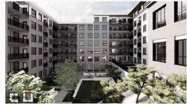
VIEW LOOKING SOUTH TOWARDS COURTYARD OF BUILDING B
