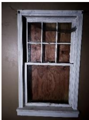
Figure 6.18 Example of existing double-hung window from the interior.
