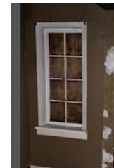
Figure 6.20 Fixed 8 pane window beside living room fireplace from interior.
