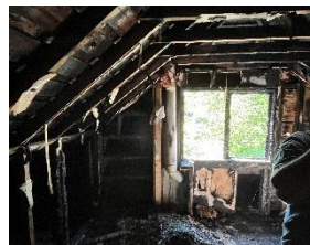
Figure 6.22 Fire damaged windows.
