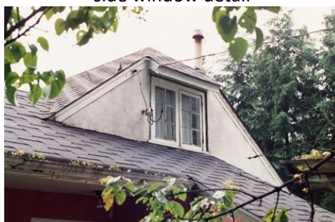
Chamfered gable and historical roof line.
