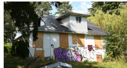
Figure 6.4 Note similar siding are applied to the second storey dormer and first storey western addition.
