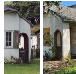
Figure 6.10 West archway and brick elements.
