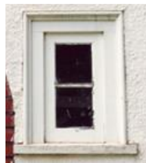
Figure 6.19 Fixed 2 pane window beside main entry door (historical photograph).
