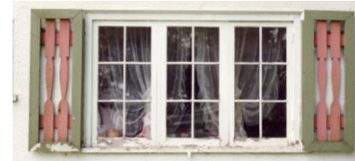
Figure 6.14 Historical shutters from archival photo collection.
