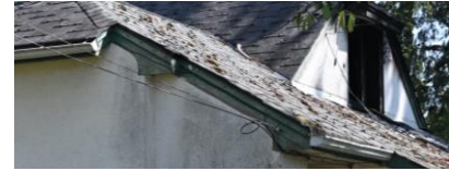
Figure 6.13 Front roof and curved box ends.
