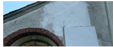
Figure 6.8 Condition of stucco
