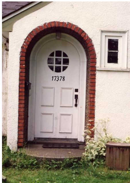
Front door and step, entry arch and side window detail
