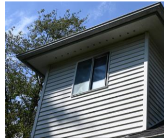
Figure 6.23 Rear dormer addition on second floor has metal sliding window.
