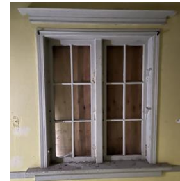
Figure 6.17 Living room 2 sash casement window from interior.
