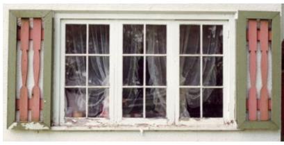
Figure 6.16 Dining room 3 sash casement window (Historical photograph)
