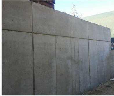
RETAINING WALL FINISH EXAMPLE:
