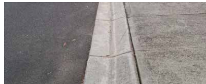
Asphalt and roll curb
