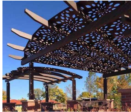
Interpretive shelter for wayfinding
