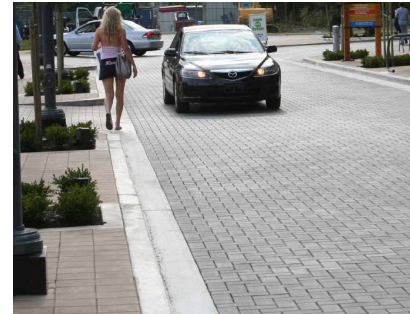
Permeable paving
