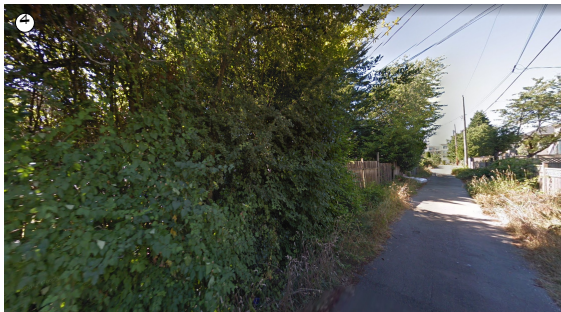
LOOKING SOUTH-EAST ALONG LANEWAY
