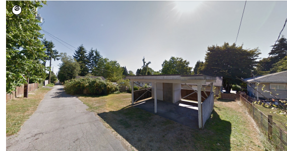
LOOKING NORTH-EAST ALONG LANEWAY
