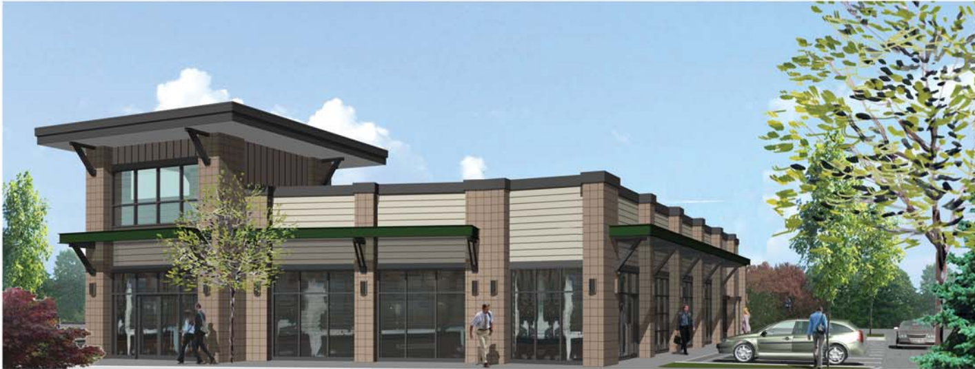
VIEW OF SOUTH WEST - BLDG. A1
