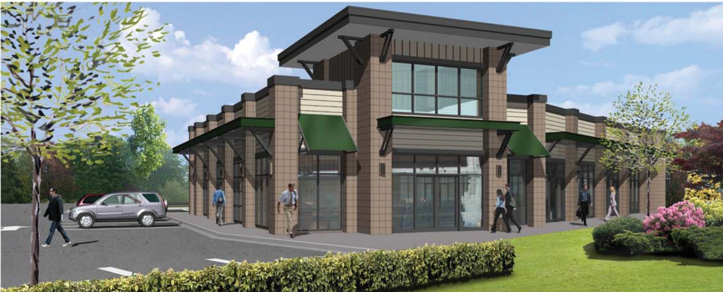
VIEW OF NORTH WEST - BLDG. A2
