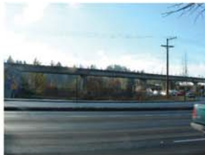
LOOKING EAST AT SITE
