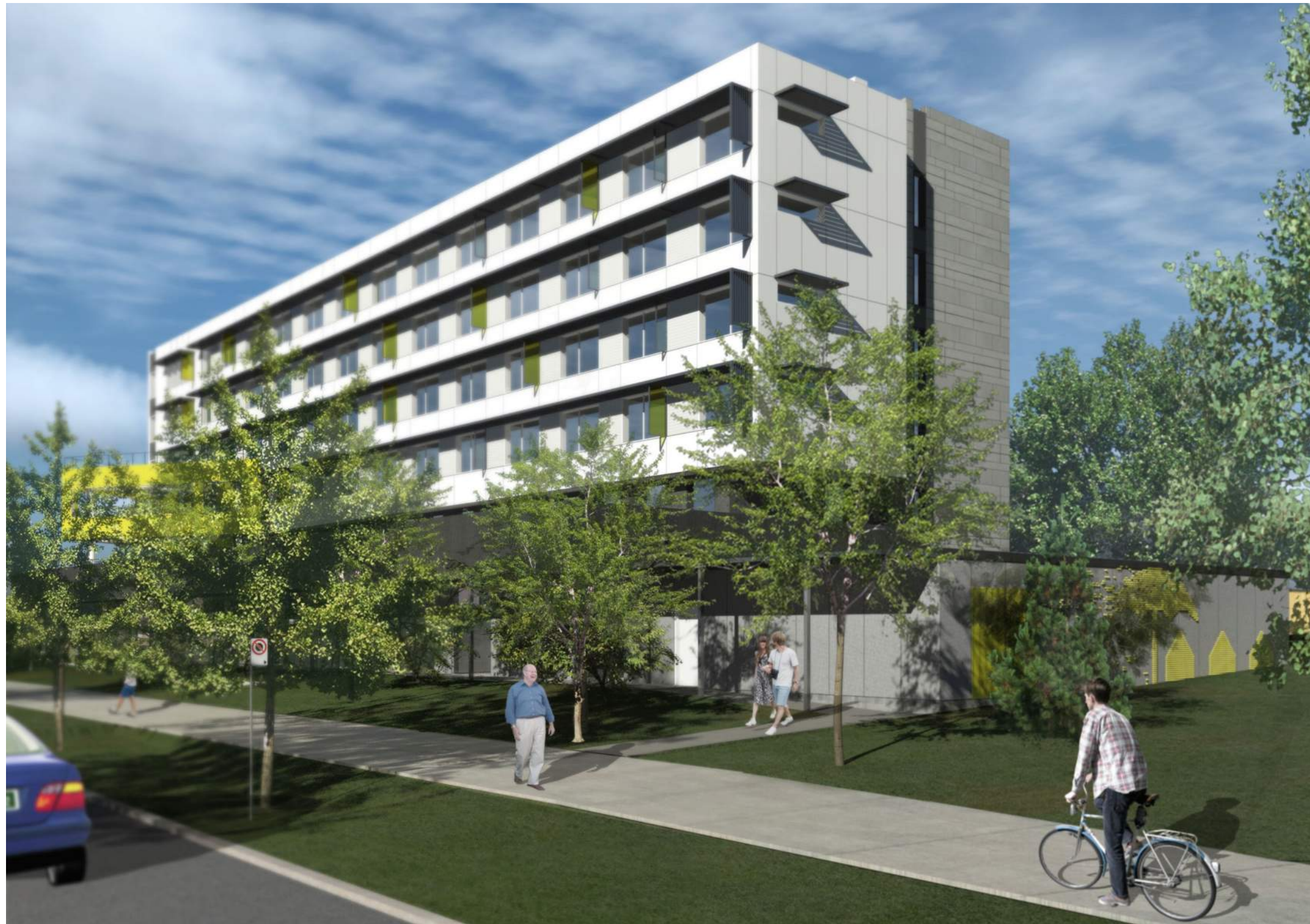
View Along Green Timbers Way Looking Northwest
