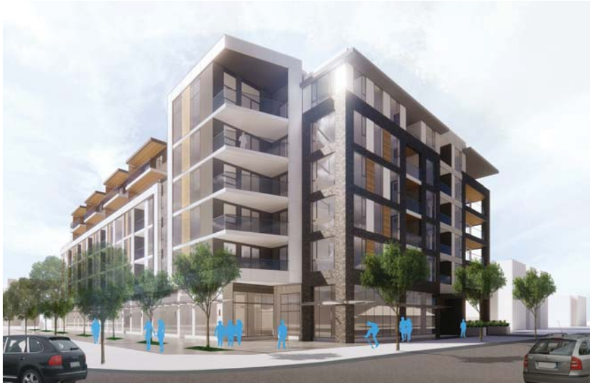
FROM THE INTERSECTION OF 152 ST. AND 19 AVE. LOOKING SOUTH WEST
