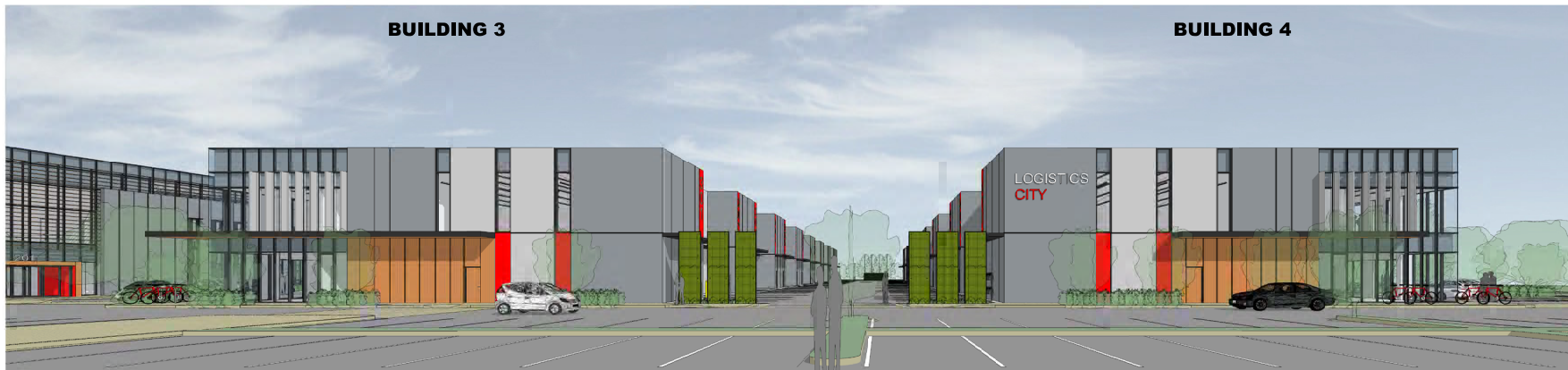
Buildings 3+4 View from West
