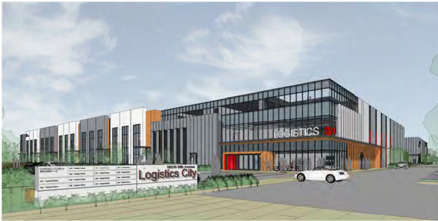
Building 1 View from North West
