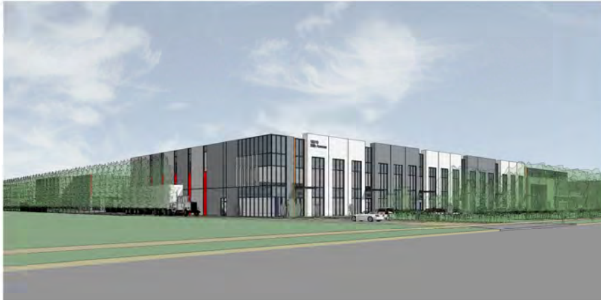
Building 1 View from North East
