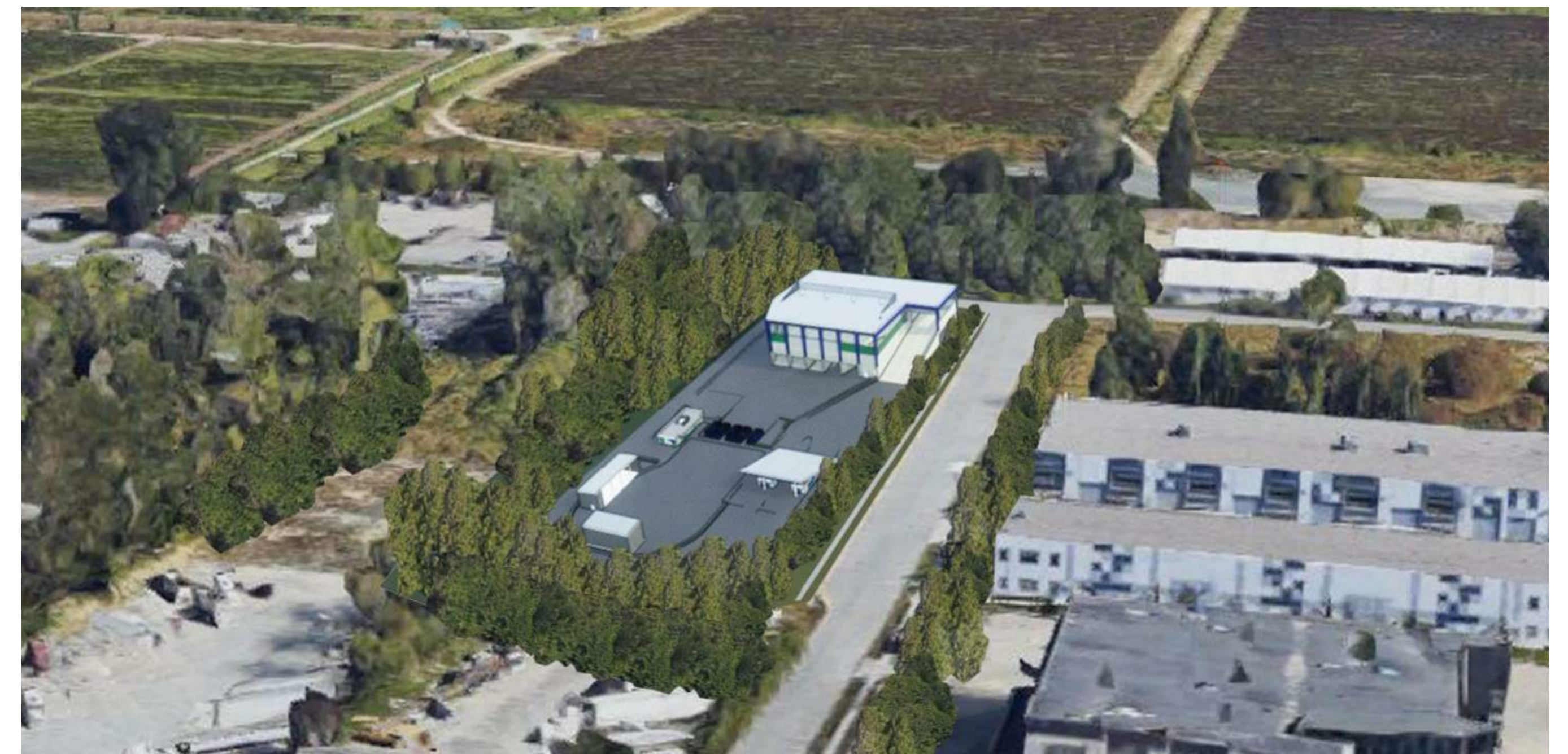
SOUTH WEST AERIAL VIEW
