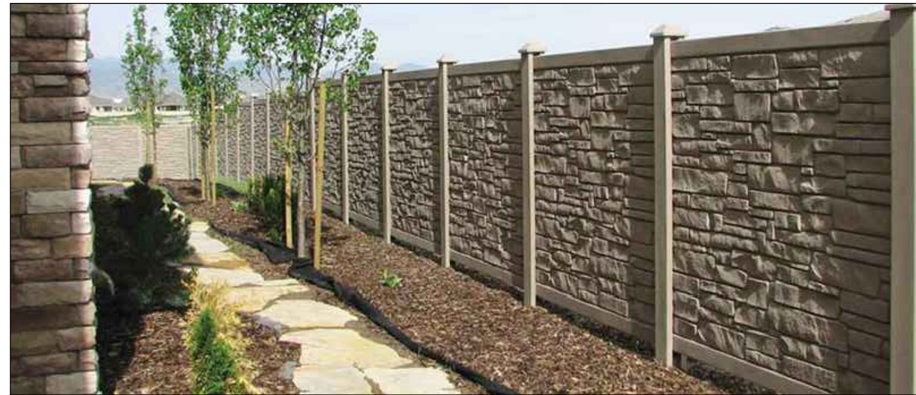
NOISE ATTENUATION FENCE
