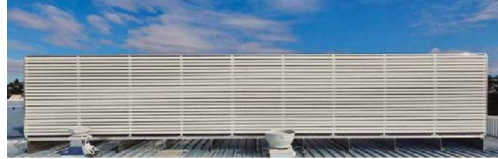
EXAMPLE PICTURE OF ROOF EQUIPMENT SCREEN*
