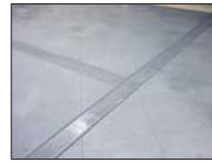
SAW CUT CONCRETE
