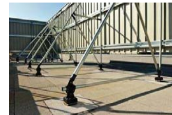
EXAMPLE PICTURE OF ROOF SCREEN BASE CONNECTION*
