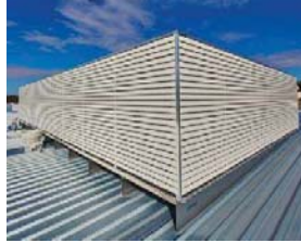
EXAMPLE PICTURE OF ROOF EQUIPMENT SCREEN*
