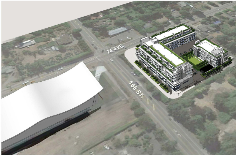
NORTH EAST AERIAL VIEW
