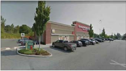
A VIEW to BLDG ABC-1
