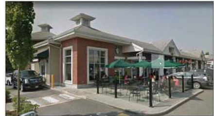
J VIEW to BLDG E-2
