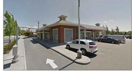
H VIEW to BLDG D-3
