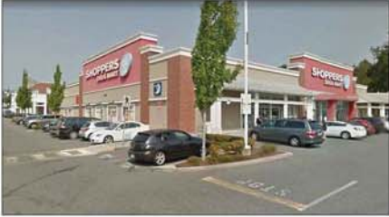
B VIEW to BLDG ABC-2
