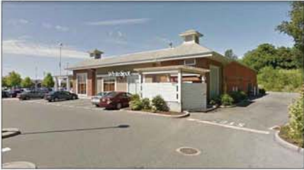
C VIEW to BLDG ABC-3
