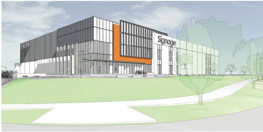
View from North East
