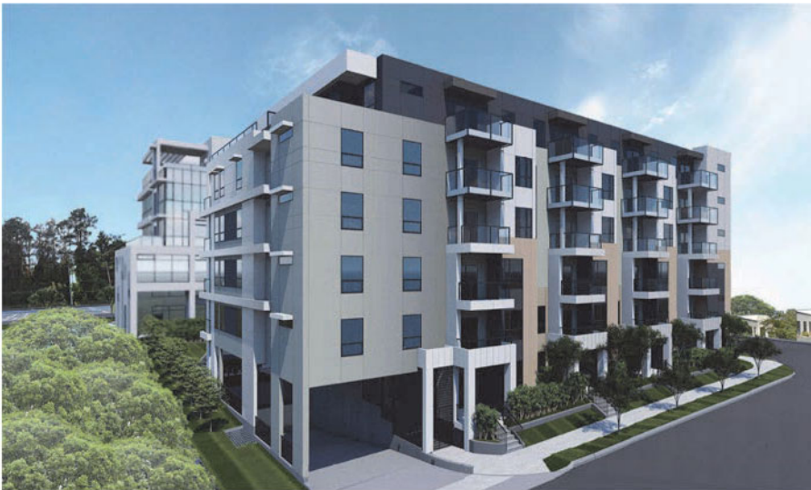
2. SOUTHEAST VIEW FROM NORTH-SOUTH LANE - RESIDENTIAL BUILDING
