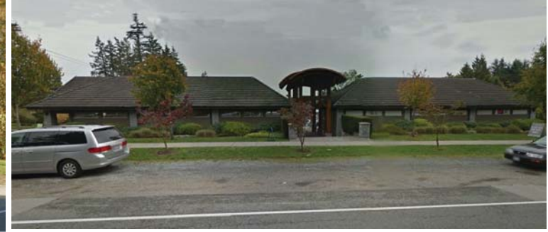
BUILDING ACROSS STREET
