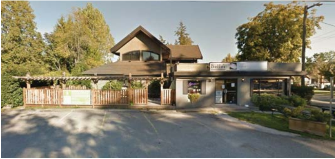
BUILDING ACROSS STREET
