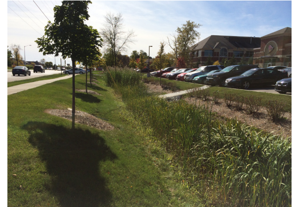
Rain garden beside a sidewalk.
