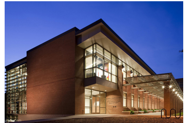
Architectural expression is integrated with building's lighting.
