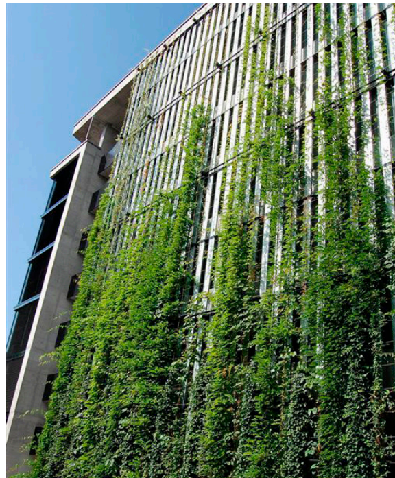
Green 'living walls' to add visual interest to buildings.
