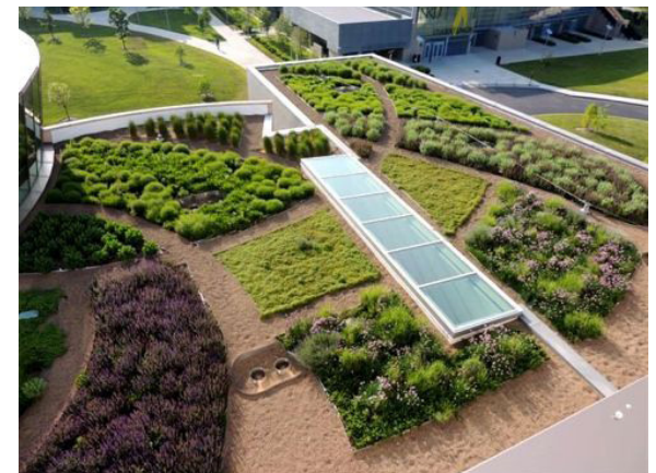
Good example of living green roofs.
