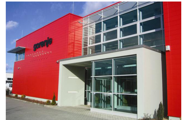
High quality materials and glazing on street facade.
