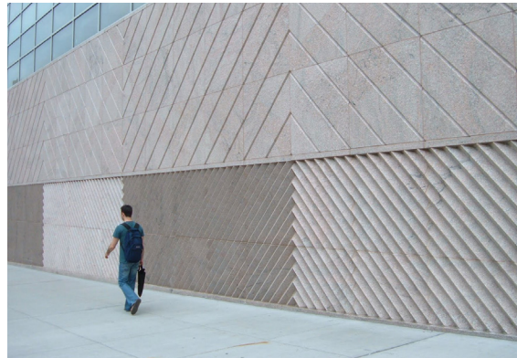
Suitable colour, pattern, texture, and finishing for blank walls and concrete facades.
