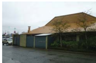
4 - BUILDING LOOKING NORTH
