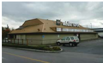
3 - BUILDING LOOKING EAST
