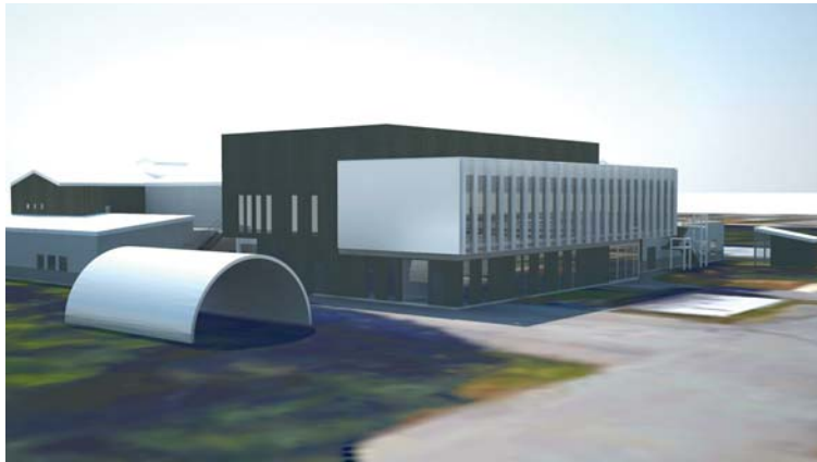
SOUTH EAST CORNER
