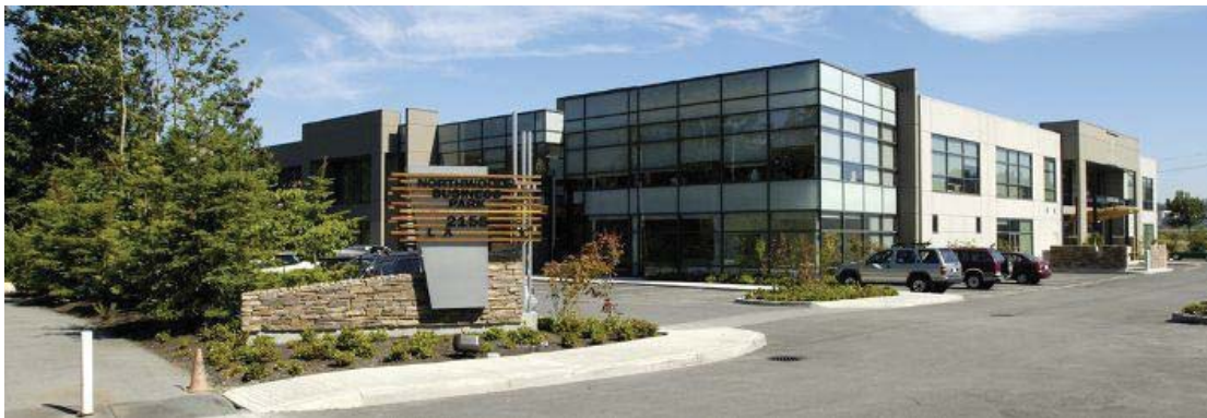
Figure 6 – High Quality Exterior Material
