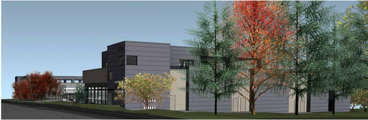
HIGHWAY 10 (56th AVENUE) STREET VIEW - DRIVING EAST
