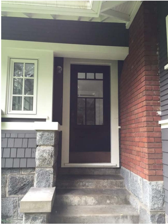
Original exterior red brick chimney
