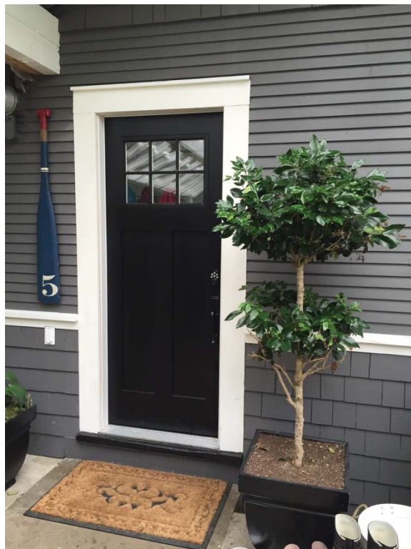
Combination of lapped and shingle cladding
