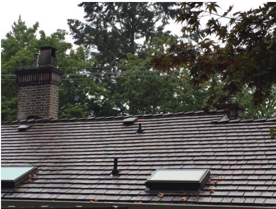
Original interior brick chimneys
