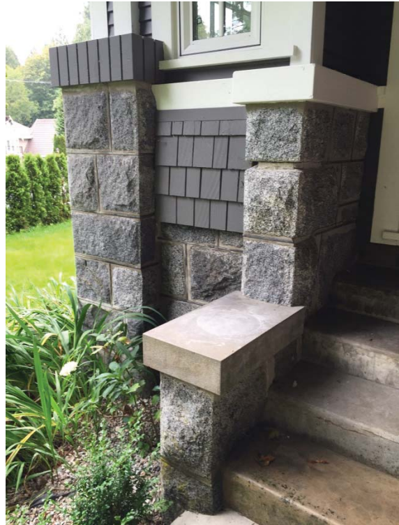
Stone (granite) foundation
