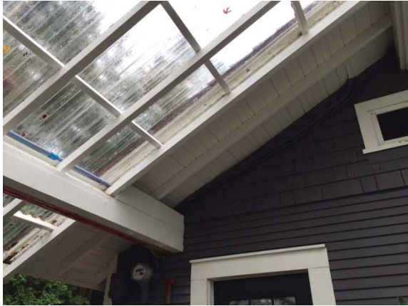
Open soffits and exposed raftertails
