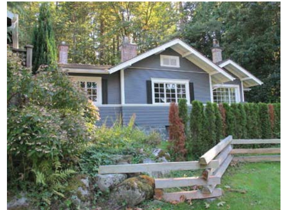
Original interior brick chimneys
