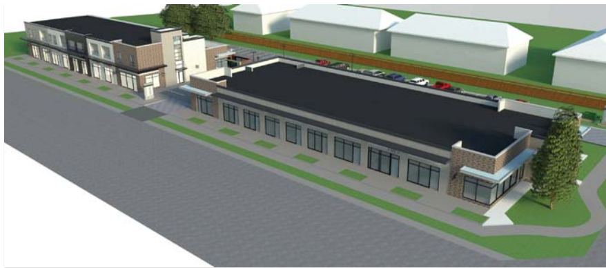
AERIAL VIEW - FROM NORTH WEST CORNER
