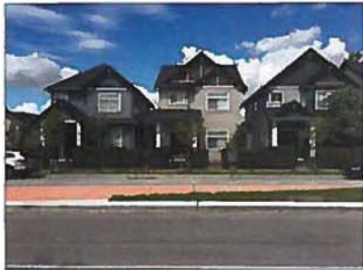
10 VIEW ACROSS STREET ON 12ND AVENUE
