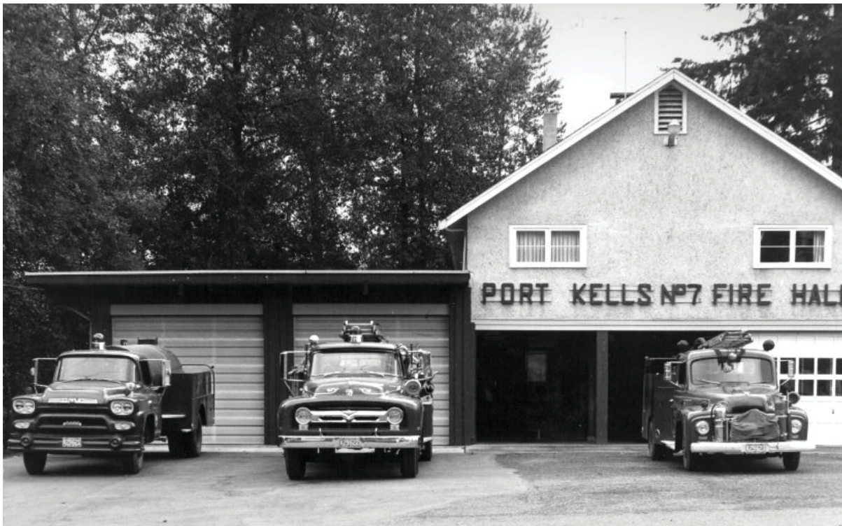
Early photograph of the Fire Hall with the original two-storey building to the right and the later addition to the left.
