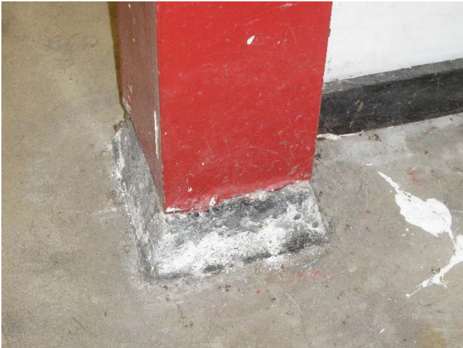
Existing 6x6 timber post supporting 3x 2x12 ceiling beams.
