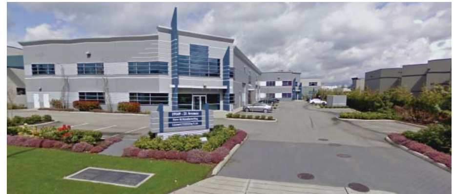
Single Driveway Access
