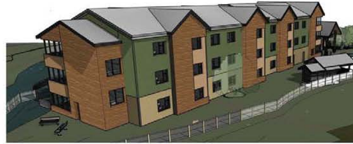
2 AERIAL VIEW - NORTH EAST
