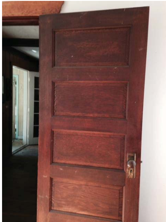
Original wood panel door and door hardware in small bedroom
