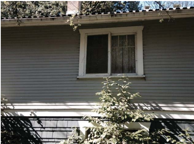
Window on east façade
