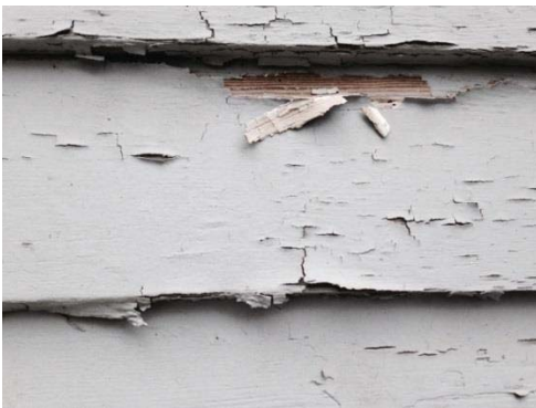
Paint scraping on weathered portion of facade
