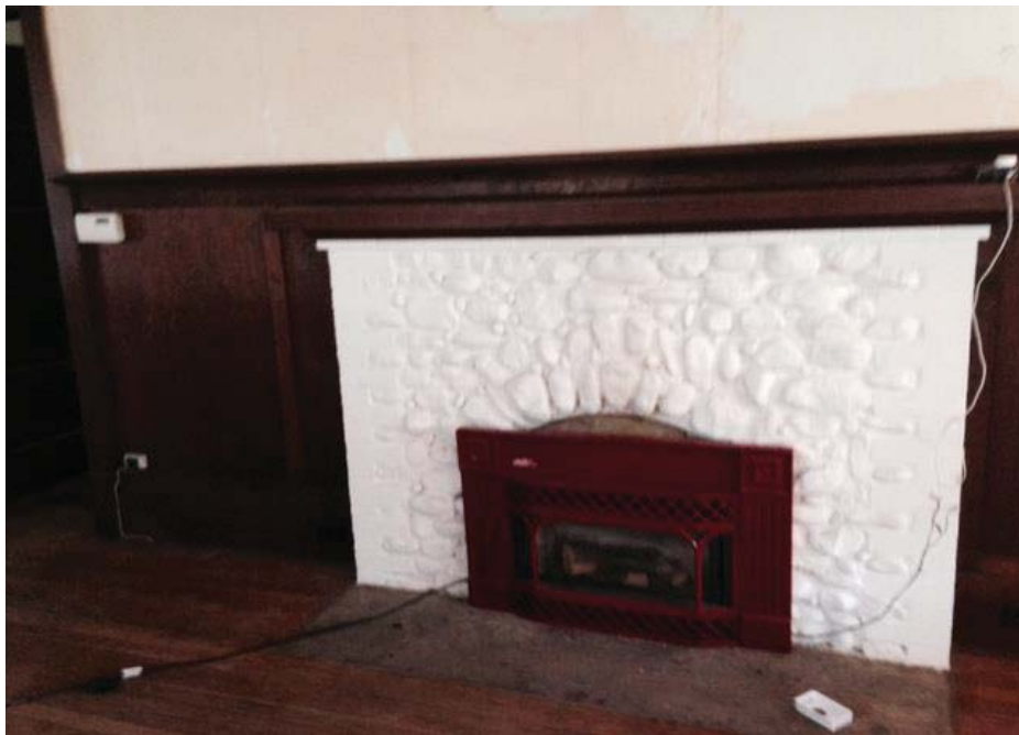
Painted pebble stone fireplace with insert and wood wainscoting in living room
