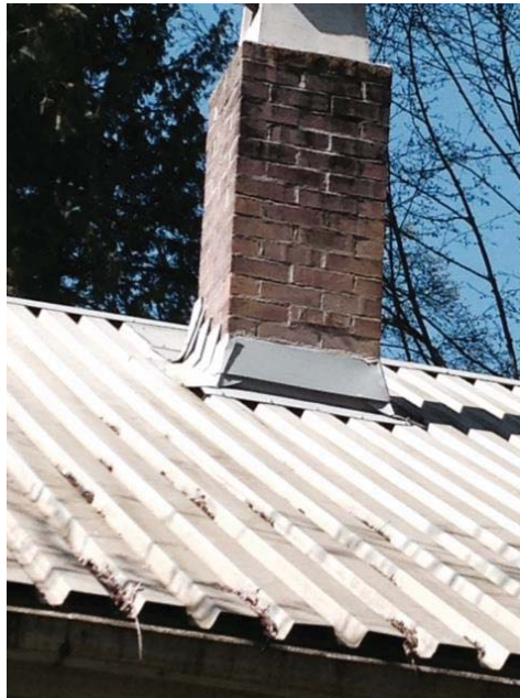
Metal roof and brick chimney
