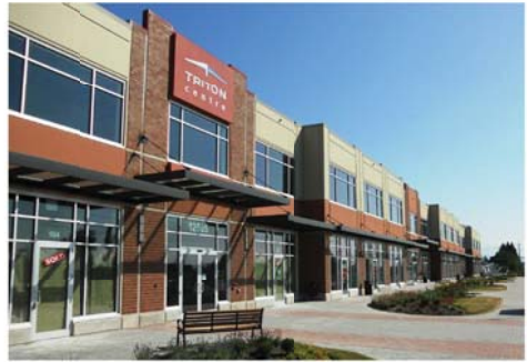
SOUTHWEST VIEW: EXISTING FRONT ELEVATION
