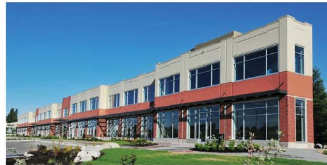
SOUTHEAST VIEW: EXISTING FRONT ELEVATION
