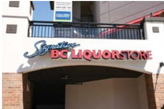
C. Large electrical raceway mounted on building fascia
