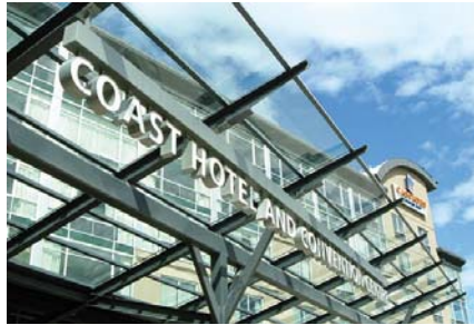
B. Letters suspended under the canopy with integrated raceway
