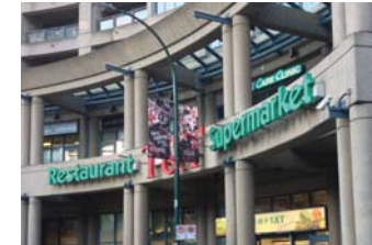
C. Signs mounted on face of canopy structure Exposed electrical supply/conduit/connections
