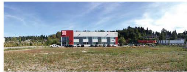
SOUTH EAST VIEW (EXISTING WILLIAMS MACHINERY BUILDING)
