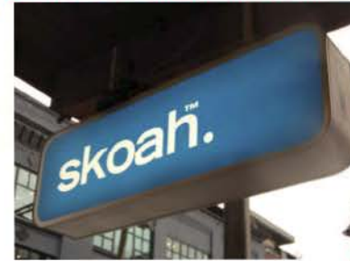
Unacceptable: Internally illuminated plastic face, back-lit sign cabinet is too thick and exposed
