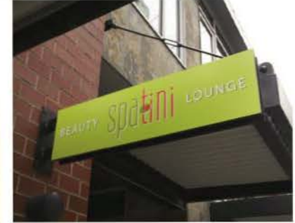
Projected sign cabinet with integral support bracket and concealed electrical supply to building fascia
