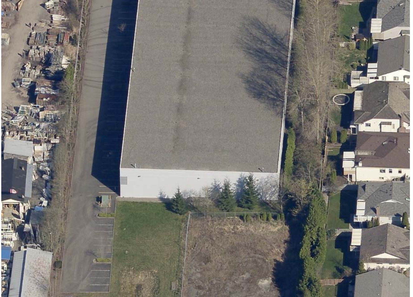
View from the South
