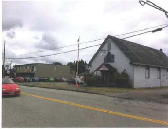
VIEW TO SOUTH EAST FROM 57TH AVENUE
