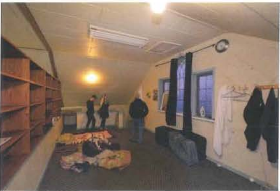
VIEW OF MEZZANINE TOWARDS STAIRS
