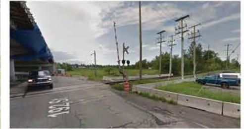
5 - VIEW OF EXISTING TRAIN TRACK AND BRIDGE LOOKING SOUTH ON 192ND STREET
