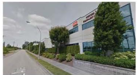
6 - VIEW OF EXISTING PROPERTY LOOKING NORTH WEST ON 52ND AVENUE
