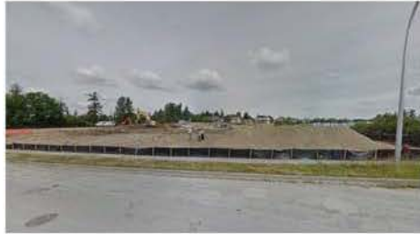
10 - VIEW OF EXISTING ADJACENT PROPERTY LOOKING NORTH ON 52ND AVENUE
