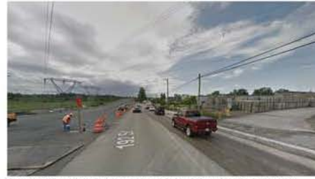
3 - VIEW OF UPGRADED ROAD LOOKING SOUTH ON 192ND ST.
