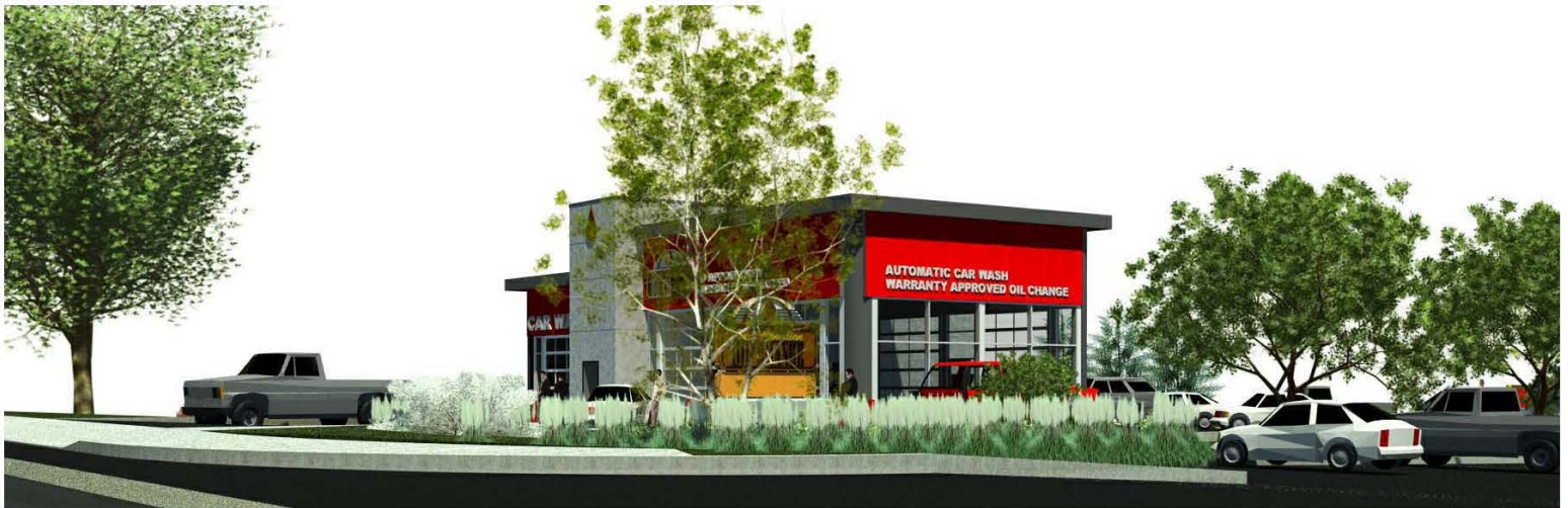
view from south west
