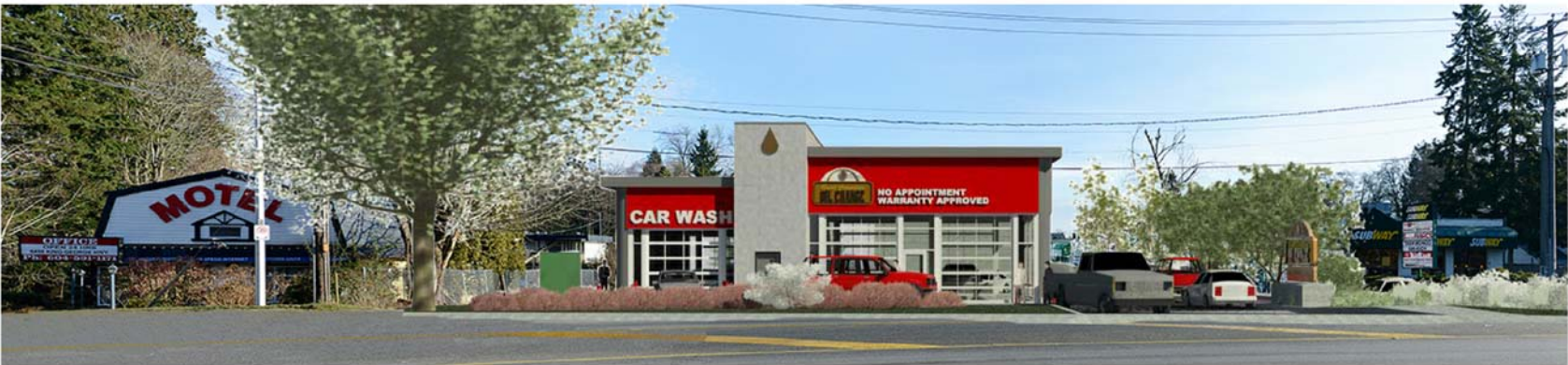
view from the west
