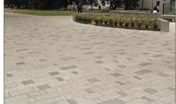
CONCRETE UNIT PAVERS ON PLAZA LANDSCAPE AMENITY AND COMMERCIAL UNIT ENTRIES
