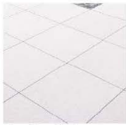
Sawcut Concrete Paving
