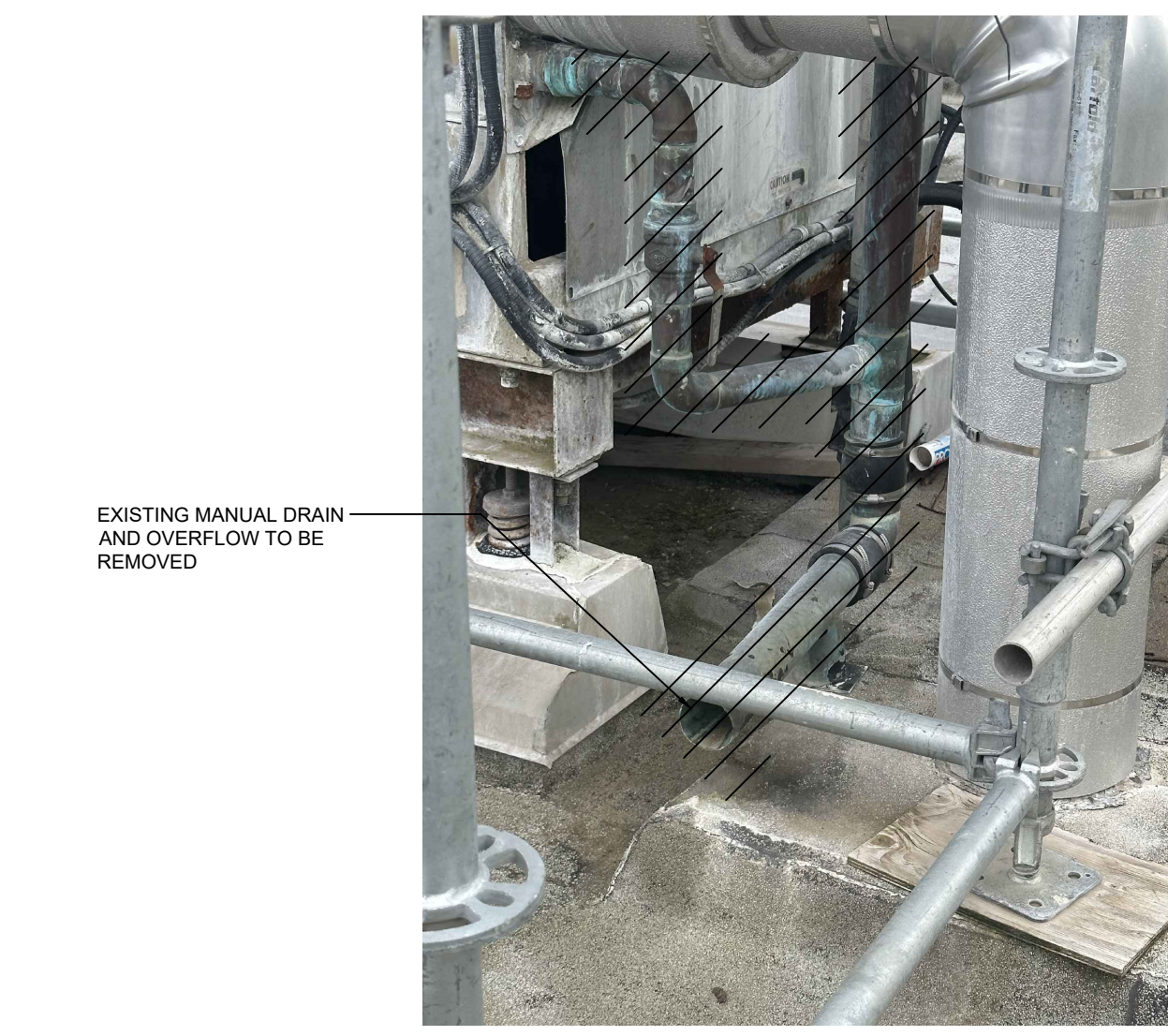
B EXISTING COOLING TOWER DRAIN M200 SCALE: 1:100
