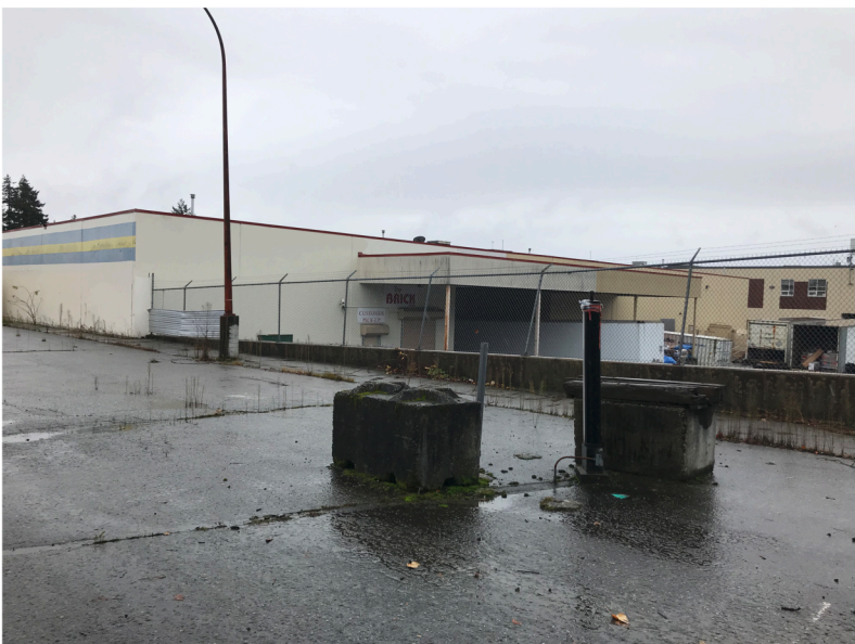
Monitoring well 2 IMG_5781.JPG
