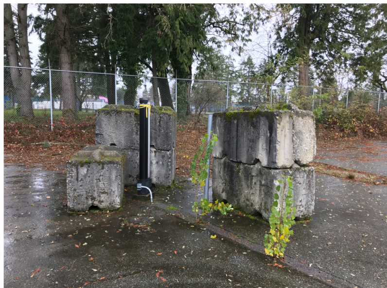
Monitoring well 3 IMG_5776.JPG
