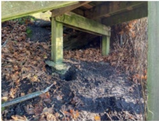
Photo 8 – Foundations under landing
