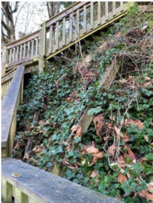
Photo 35 – Braces between stairs sections
