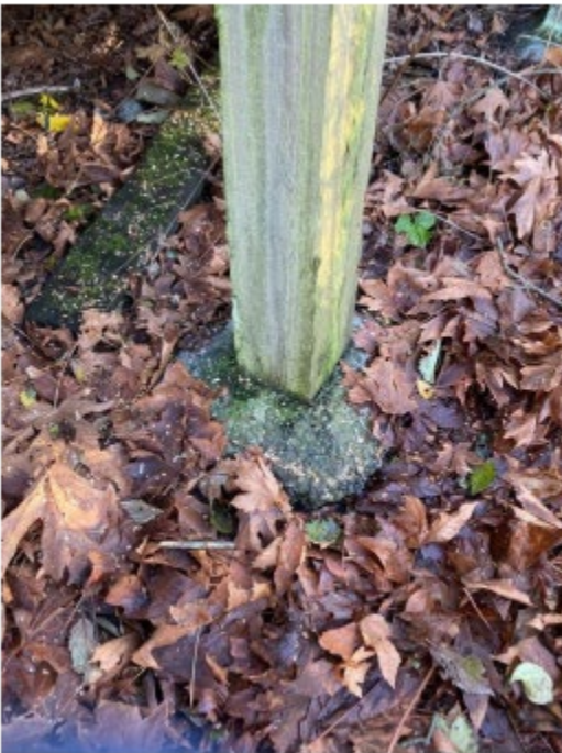
Photo 7 – Typical concrete foundation
