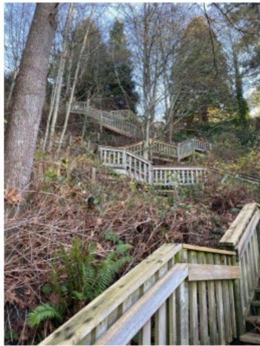
Photo 2 – View halfway up stairs
