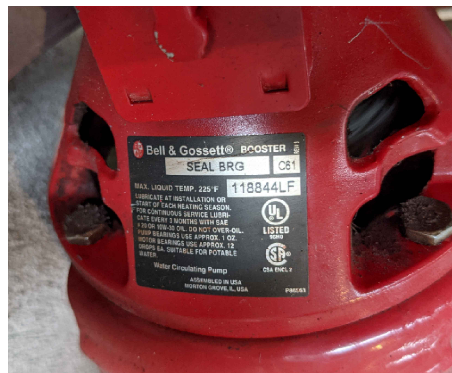
5 EXISTING DHWR PUMP (P-DHWR) SCALE: NTS
