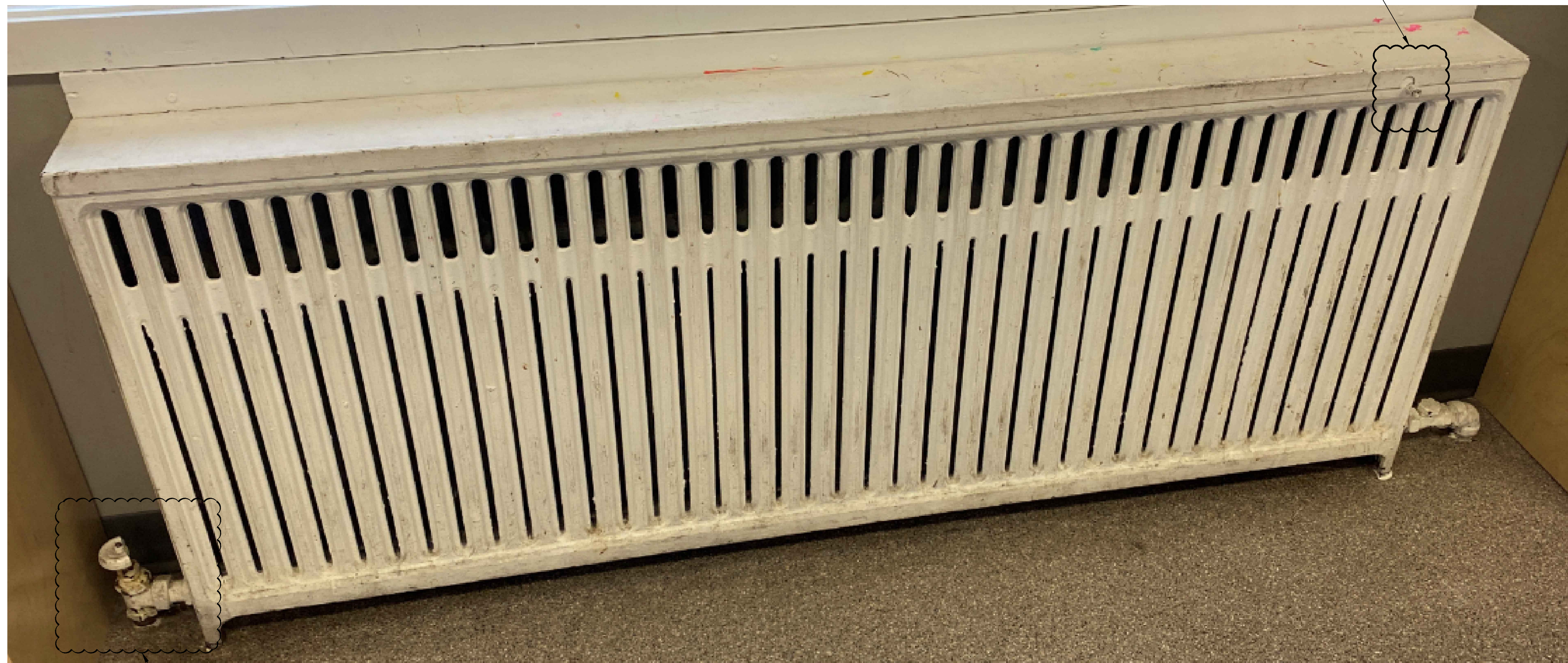
1 EXISTING BOARDROOM CAST IRON RADIATORS M1.05 SCALE: NTS
