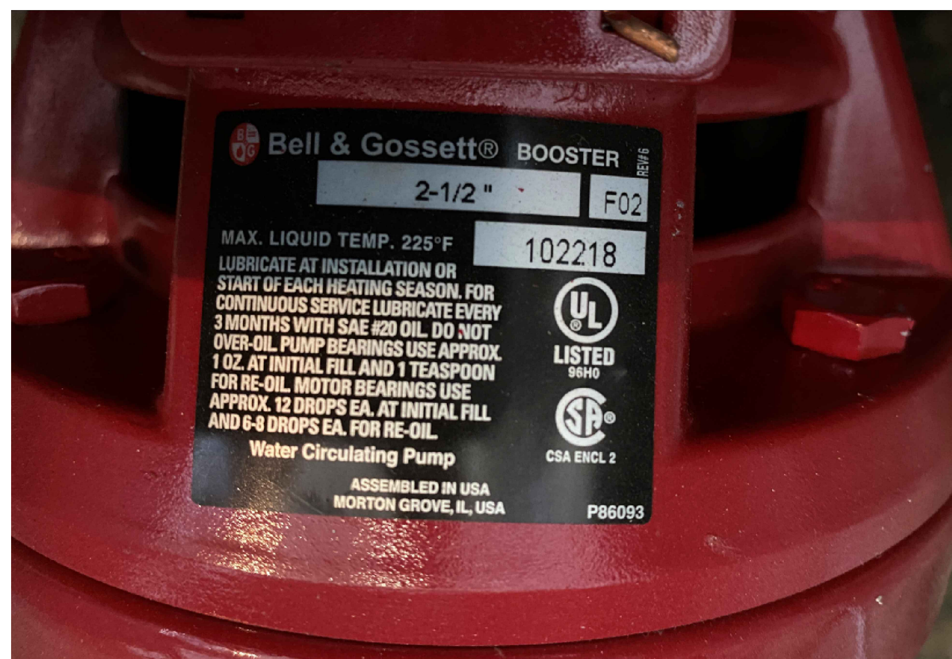
4 EXISTING BOILER CIRCULATION PUMP (P1/BRDRM_PMP & P2/HALL_PMP) SCALE: NTS
