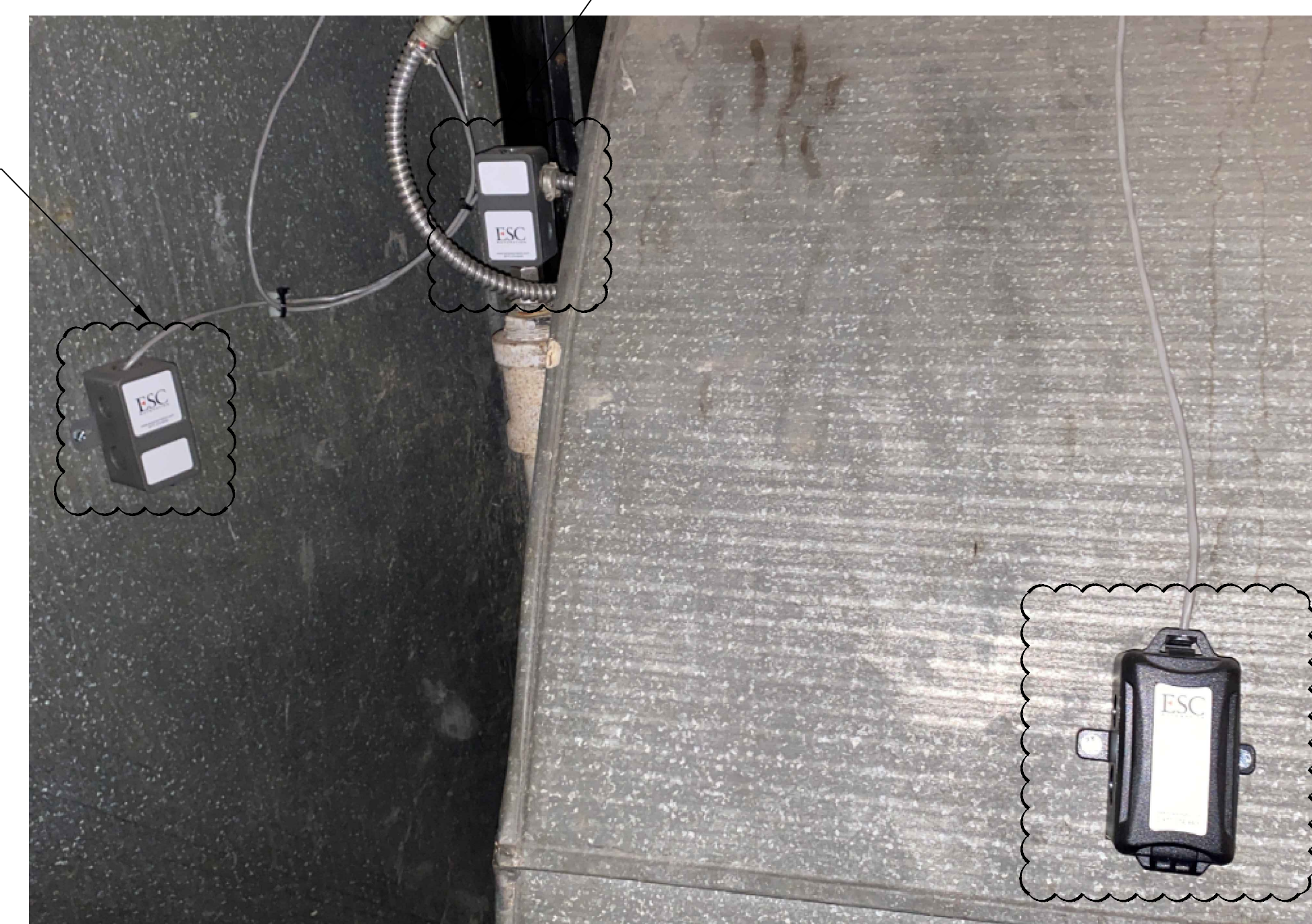
4 EXISTING FAN COIL ROOM TEMPERATURE SENSORS SCALE: NTS
