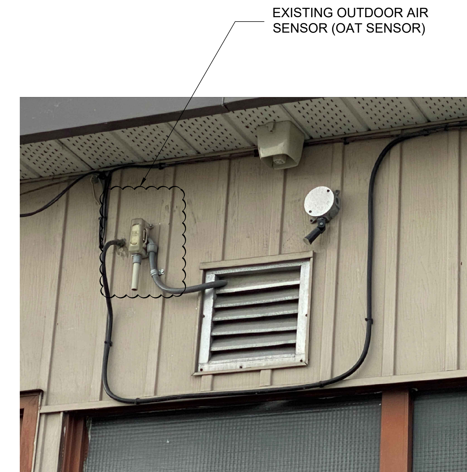
6 EXISTING O/A TEMPERATURE SENSOR (OAT SENSOR) SCALE: NTS
