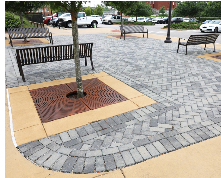
Top Image: Example of a warehouse constructed from mass timber in Langford, BC. Bottom Image: An example of a public plaza that incorporates permeable paving and shade trees to provide a comfortable environment for people, while promoting storm water infiltration.
