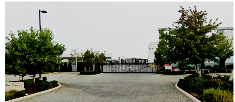
Top: an illustrative example of how site planning should be the primary mitigating measure for security and how that if required, security fencing should be sited away from public streets. Bottom: an example of low height and visually unobtrusive security fencing.
