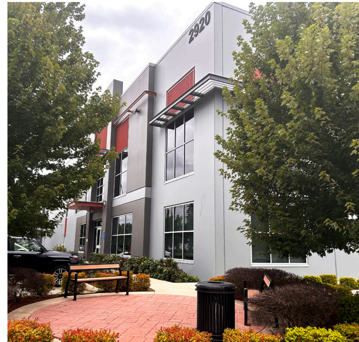
Top right and bottom right: Examples of well landscaped employee amenities.
